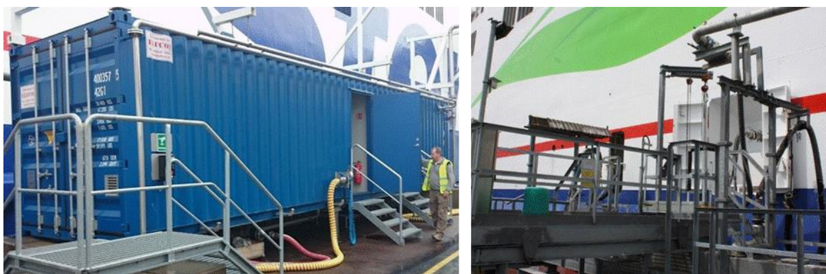
Figure 16: Stena Germanica bunker station enclosure (left photo) and platform for hose connection (right photo). The bunker hose is connected to the ship's system using drip-free connections. (Photos: J. Ellis)
