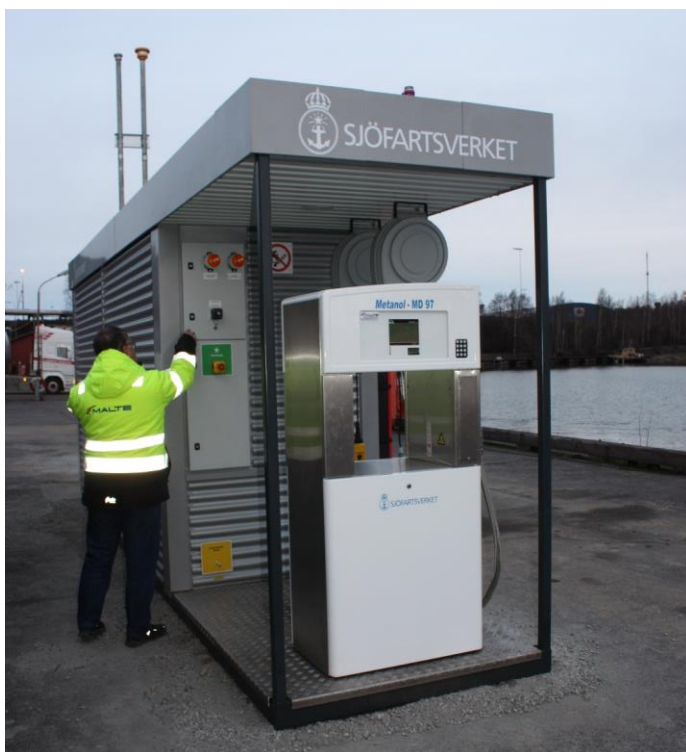
Figure 17. Methanol (M97) refuelling facility at the Swedish Maritime Administration's Oxelösund pilot boat (Photo: J.Ellis)
